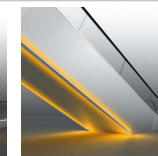
Side and soffit cladding
