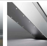
Soffit LED spotlighting
